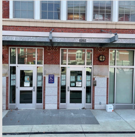
3rd, 4th, & 5th Grades/Grado Main Entrance Entrada Principal (17th St.)
