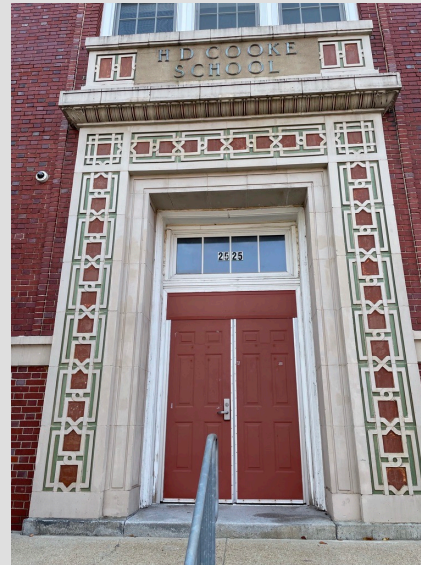
1st Grade/ 1er Grado Original Main Doors/ Puerta de Entrada Original (17th St.)
